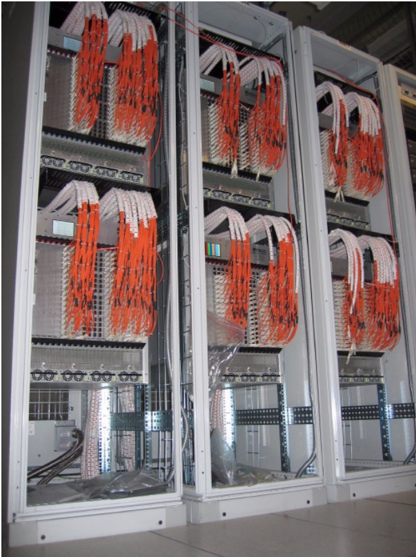
The 3 racks containing the 6 Myrinet switches used to collect the data from the FRLs.
