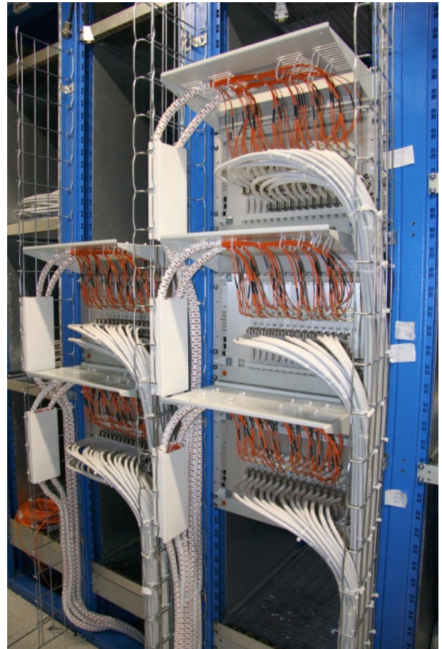
One of the 15 racks containing the FRL cards. In gray, the s-link cables and in orange, the optical patch cords.
